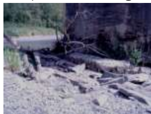
North Side of Pier 4, August 30, 2010
