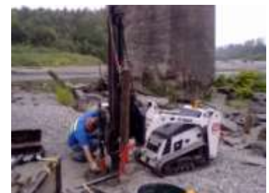
Drilling at Haller Trestle, Pier 4
