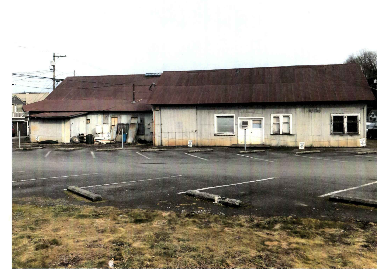
EXISTING CONDITION @ PARKING AREA
