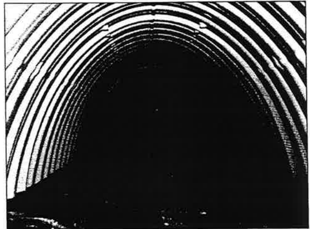
Looking down the Isolator Row.
