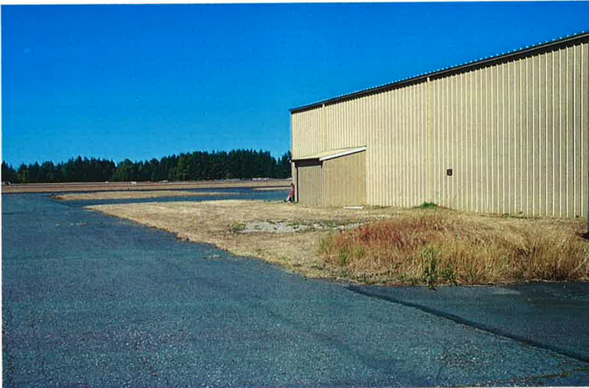
Infiltration Basin Area for Phase 2 W viewing to the West
