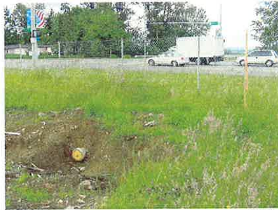
VIEW 2: Looking south-west at existing SS stub.
