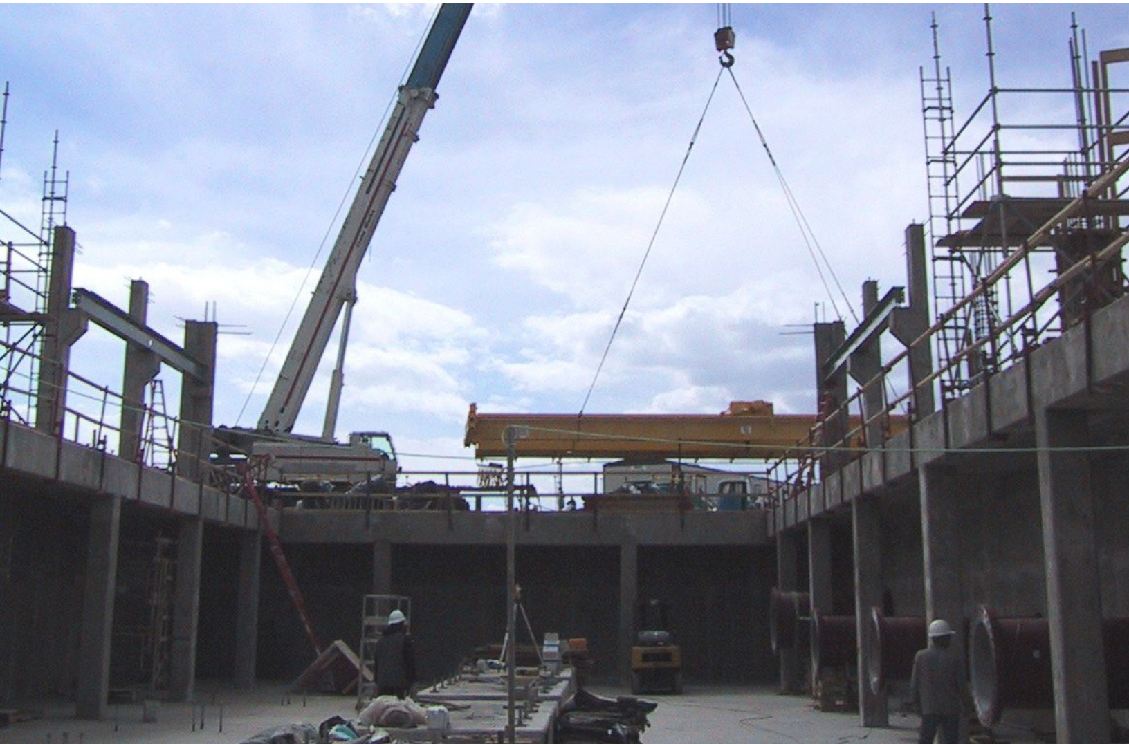
Twin Rock Pump Station Design-Build
