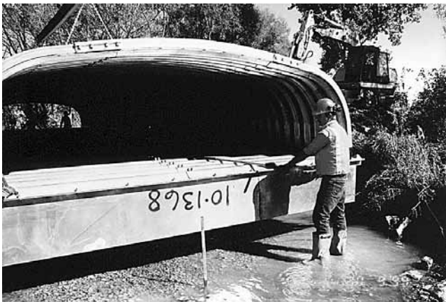
Installation of Aluminum Box Culvert Toewall
