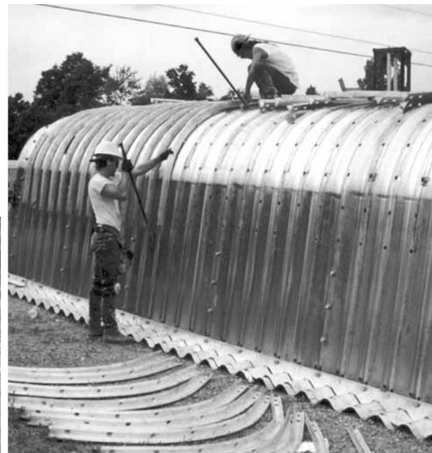
Installation of Ribs
