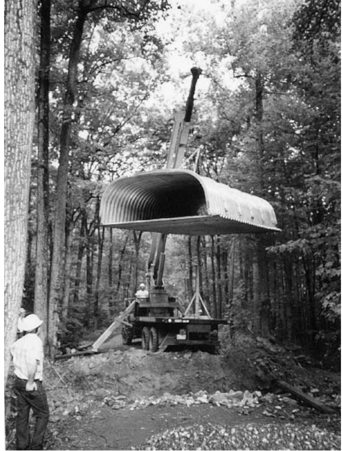
Lifting of Aluminum Box Culvert
