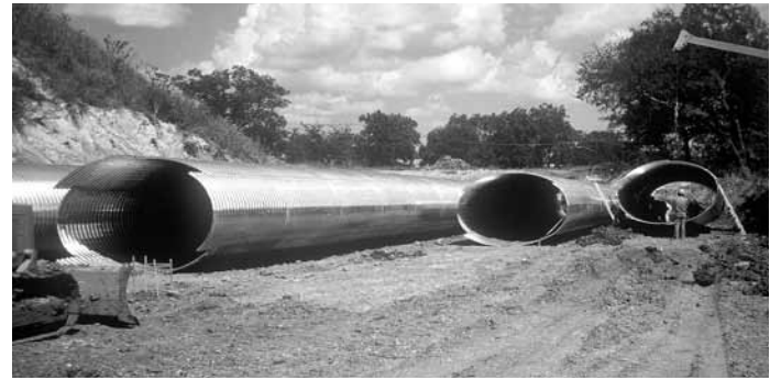
Installation of Aluminum Horizontal Ellipses
