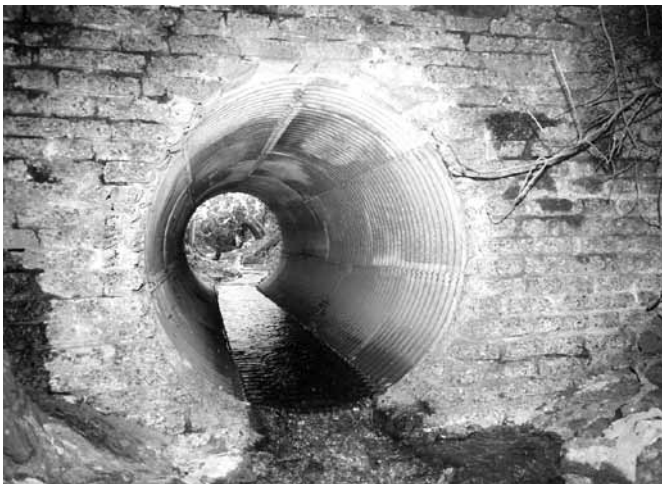
Steel Structural Plate Installed in 1946 Inspected in 1998
