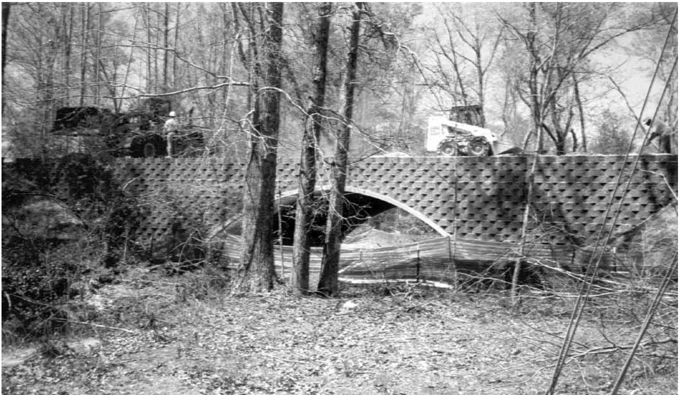
Aluminum Structural Plate Single Radius Arch with KeyStone Headwalls for Wetland Crossings
