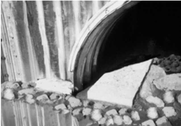
Protect footings from scour
