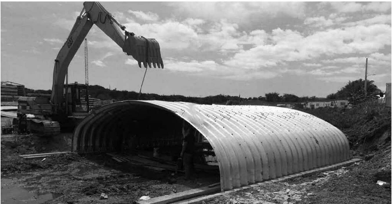
BridgeCor box culvert in Puerto Rico
