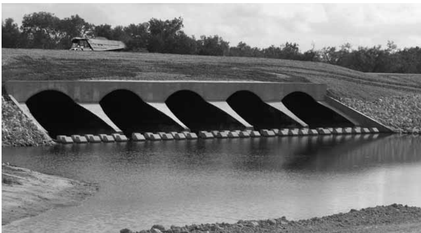
Grade Separation Structure
