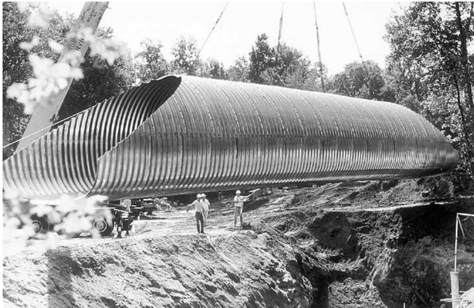
Lifting of Aluminum Pipe Arch
