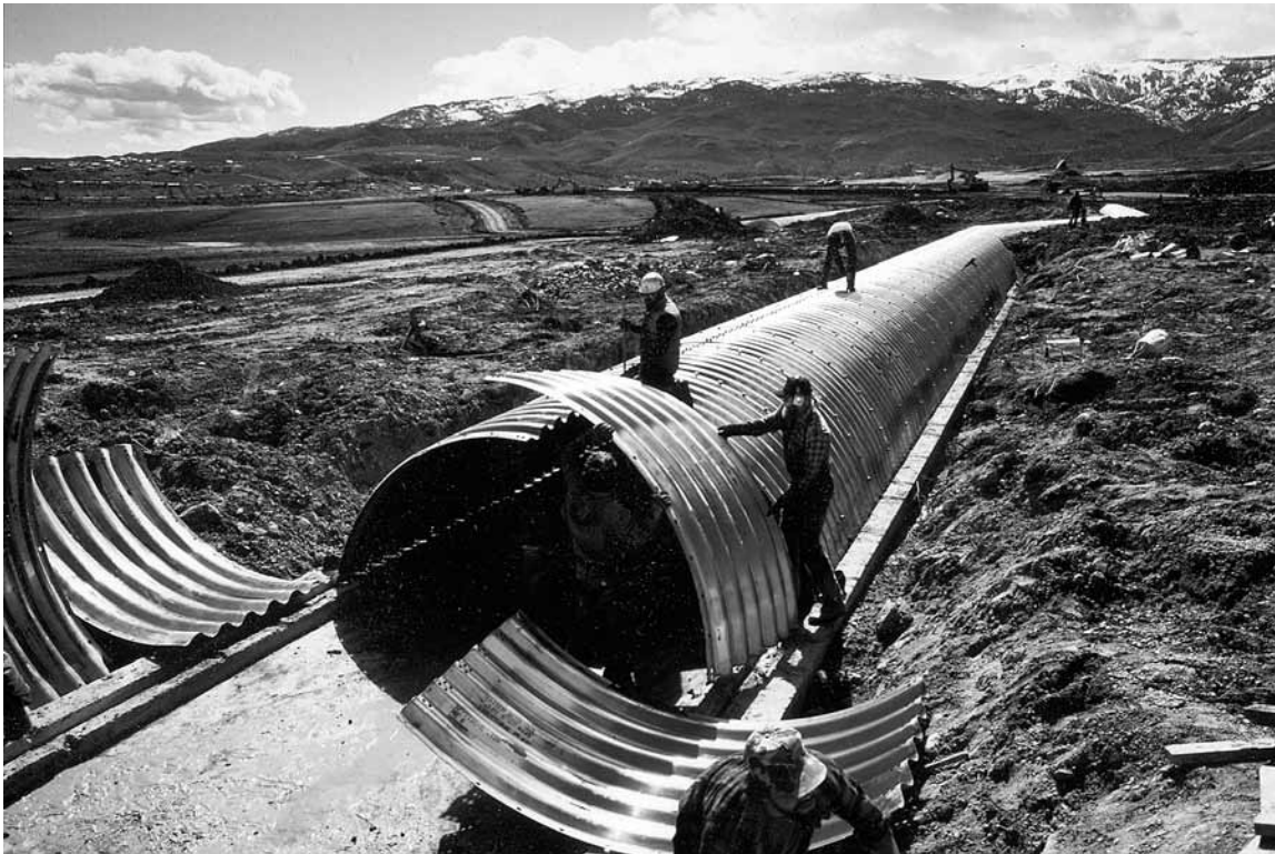
Assembly of Aluminum Structural Plate Single Radius Arch
