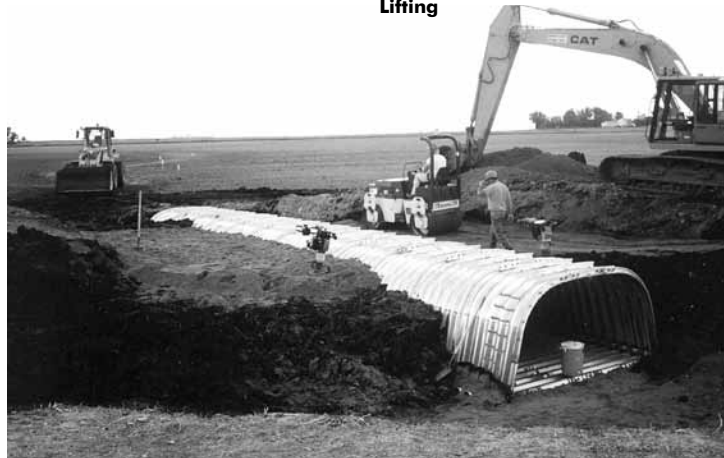
Backfill Operation
