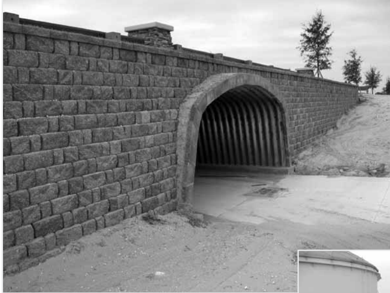
Aluminum Box Culvert Pedestrian Underpass
