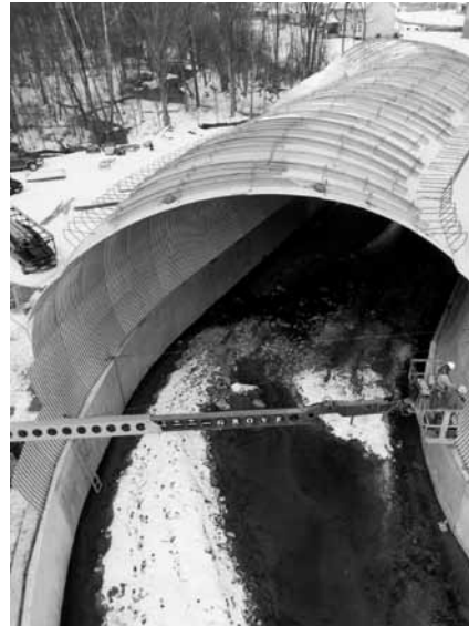
SUPER-SPAN structure near Hamilton, Ohio
